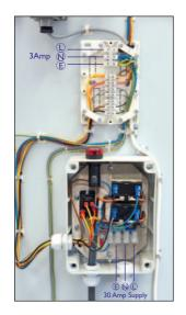
The higher immersion heater can be wired to a 15 amp switched spur for the householder to use as boost during periods of heavy hot water demand.
